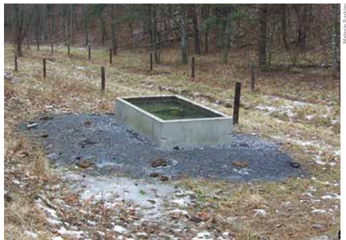
This spring development collects water in a wet area. The system uses a collection tank that fills a watering trough. This type of system can also include frost-free water hydrants that use gravity to provide water in other areas of the pasture.
