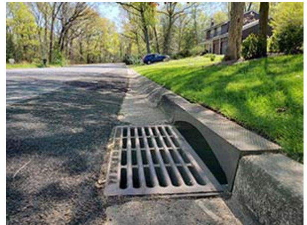
Figure 4. A storm drain in a residential neighborhood in Upper Deerfield, NJ. Stormwater runoff from the road and residences is collected by the storm drain. In this case, the runoff then flows by underground pipe to a nearby detention basin.
