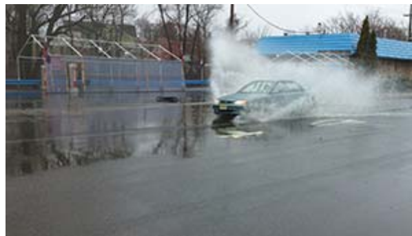
Figure 2. Unmanaged stormwater can lead to localized flooding and hazardous driving conditions, as seen on this road in Paterson, NJ.
