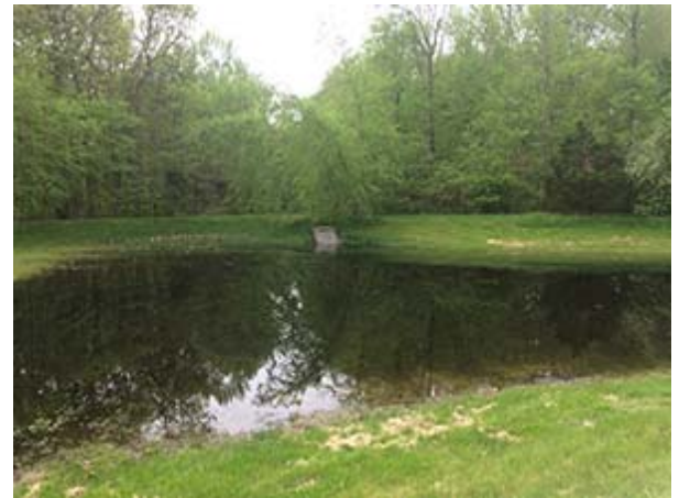
Figure 6. A stormwater detention basin in a residential neighborhood in East Windsor, NJ. An overflow structure is located in the background center. Improperly functioning detention basins can have standing water that can lead to further flooding and mosquito breeding areas. The bottom and sides of the basin are maintained as mowed turf.
