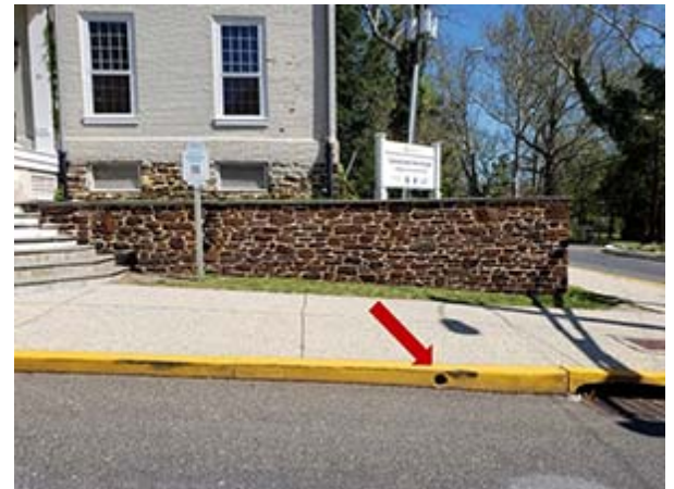
Figure 5. In some urban and suburban settings, stormwater runoff from building roofs is collected by downspouts and piped below the lawn and sidewalks to the street. Here, the outlet to the street is the round hole in the yellow curb to the left of the storm drain on the road. In these cases, stormwater from the roof passes to the municipal stormwater system without being detained or absorbed by the lawn. Rutgers Cousteau Center in Bridgeton, NJ.
