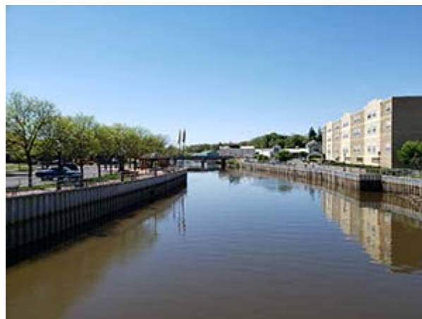
Figure 3. Some urban areas are built along rivers so that stormwater runoff flows directly to the river without intervening detention basins or green infrastructure. Here, outfall pipes for stormwater can be seen in the flood walls. The Cohansey River in downtown Bridgeton, NJ.
