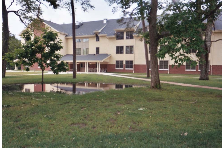
Figure 2: Water ponding on the surface of the lawn can show compacted soils that are inhibiting infiltration back into the ground. (Photo Credit: Michael Gross)
