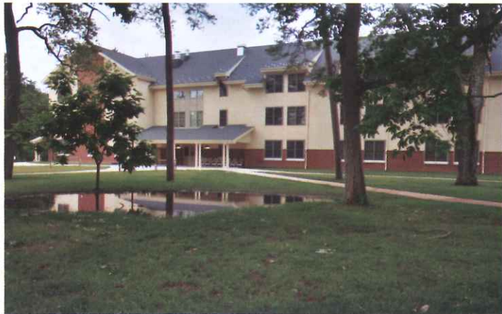
Figure 2: Water ponding on the surface of the lawn can show compacted soils that are inhibiting infiltration back into the ground. (Photo Credit: Michael Gross)
